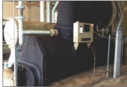
New insulation installed
