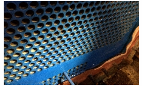
Same tubesheet opened for annual inspection, no defects were found
